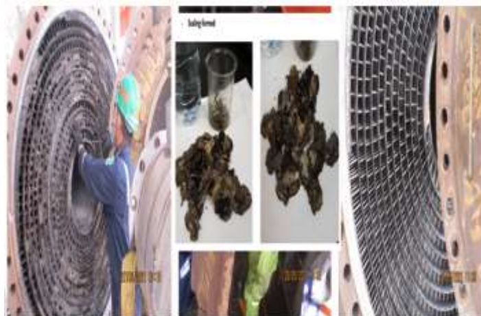
Figure 8. Inspect and clean up Reclaimer Loop Heater
