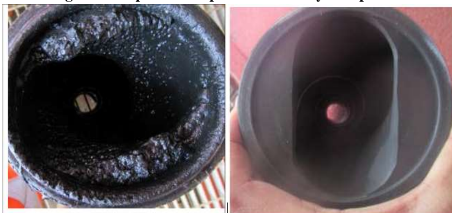
Figure 9. Inspect and replaced the Slurry Pump stator
