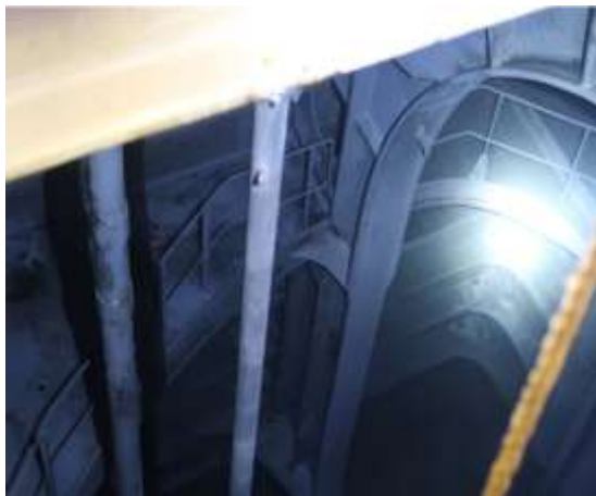
Figure 7. Inspect and clean up Rich MEG Tank
