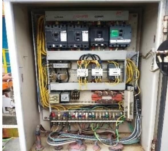
**Gambar 1** Panel *hoist crane*
