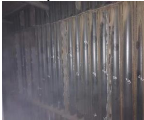
Figure 10. Installed grid in Sumsel-5
