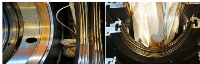
Figure 3. Oil deflector replacement and clearance adjustment
