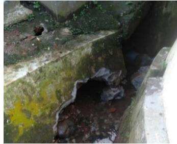
Gambar 4. Pipa Pecah
