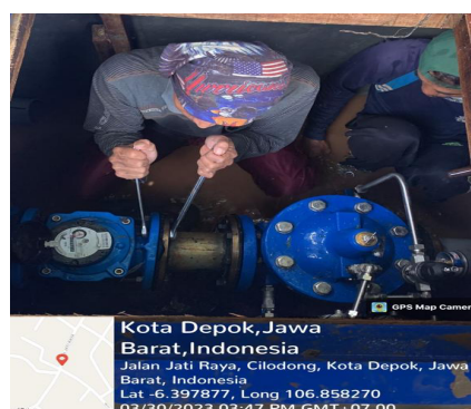
Gambar 9. Pemasangan PRV ( Pressure Reducing Valve )
