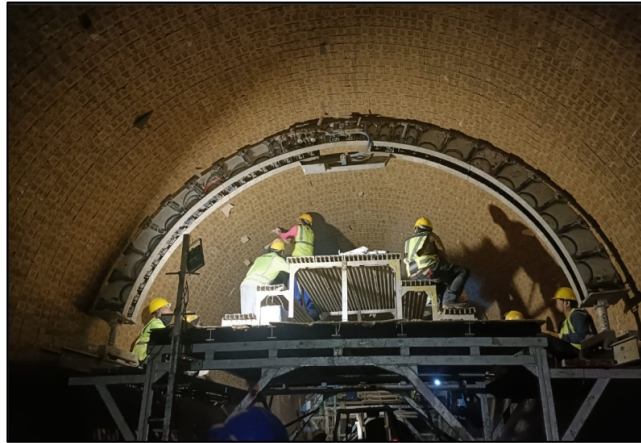
Gambar 17. Kiln Refractory installation
