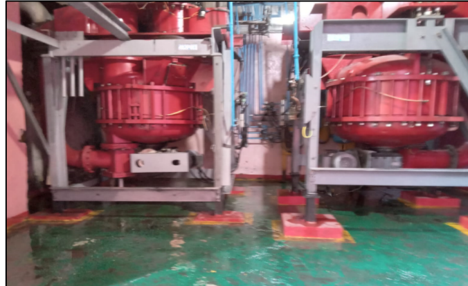
Gambar 4. Pulfurized Coal Weight Feeder
